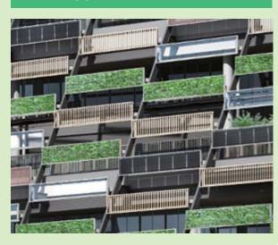
Eco-veil is composed of 741 solar electricity generation panels for city office with maximum power of 57kw., and green panels, etc.
